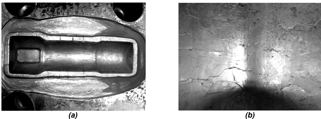
Fig. 1. Cracks on the forging die: a) die view; b) cracks on forging die surface (detail)
